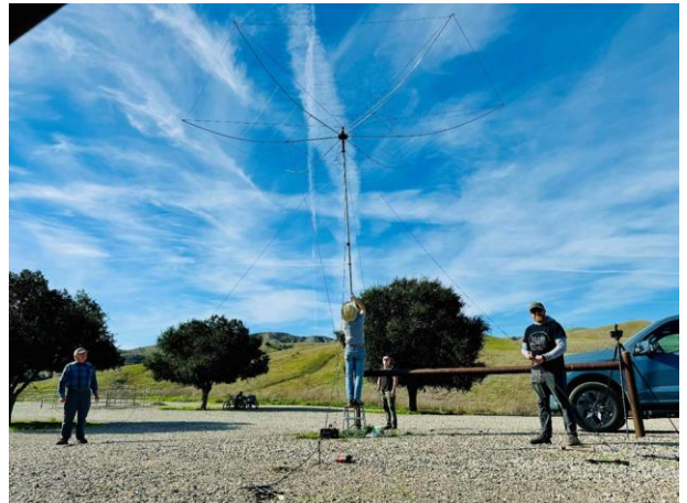
Masting a triband hex beam provided by Chris N6FR, with support from Josh KI6NAZ, Bill W6QR, and new club member Barclay K6BDO. Photo by Mark KD7DTS
